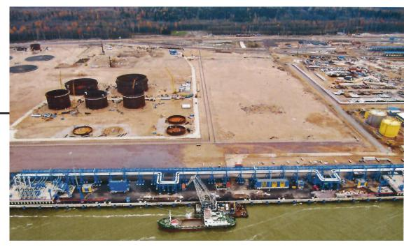
dock wall with metal sheets at depths ranging from 4 to 17.5 meters. The dredging continued all winter long, with cold weather and ice conditions at the port greatly hampering the mostly underwater work.
